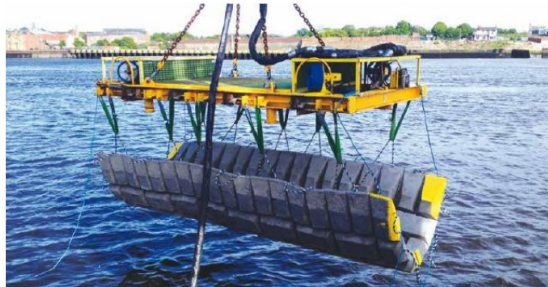
Figure 7 Indicative ROV Mattress Deployment Frame
